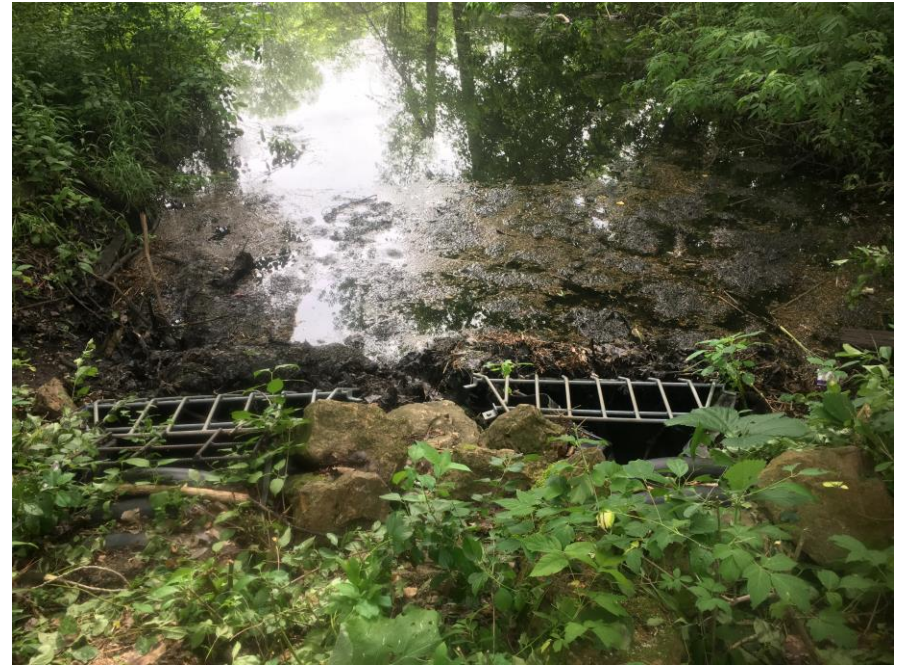
Upstream side of culvert
